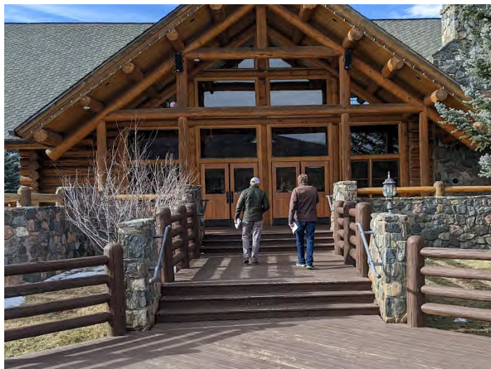
2. Deck does not have ramp to lower area
