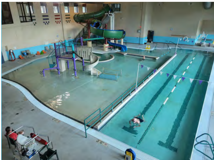
5. Pool and pool deck as seen from entry level
