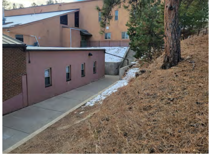
8. Area on west side for potential expansion
