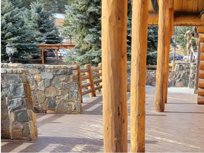
1. Guardrails in need of repair
