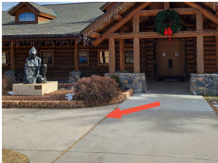
1. Settling and separation of sidewalks
