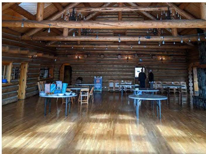
5. Wood floor at end of serviceable life
