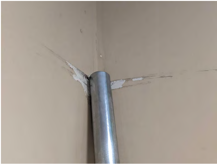
3. Drywall damage
